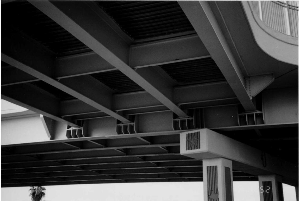
**Figure 60** Framing of an elevated T-intersection steel girder bridge in McAllen, TX. The intersecting span is supported on a series of steel corbels formed of partial depth stiffeners with a cap plate.
