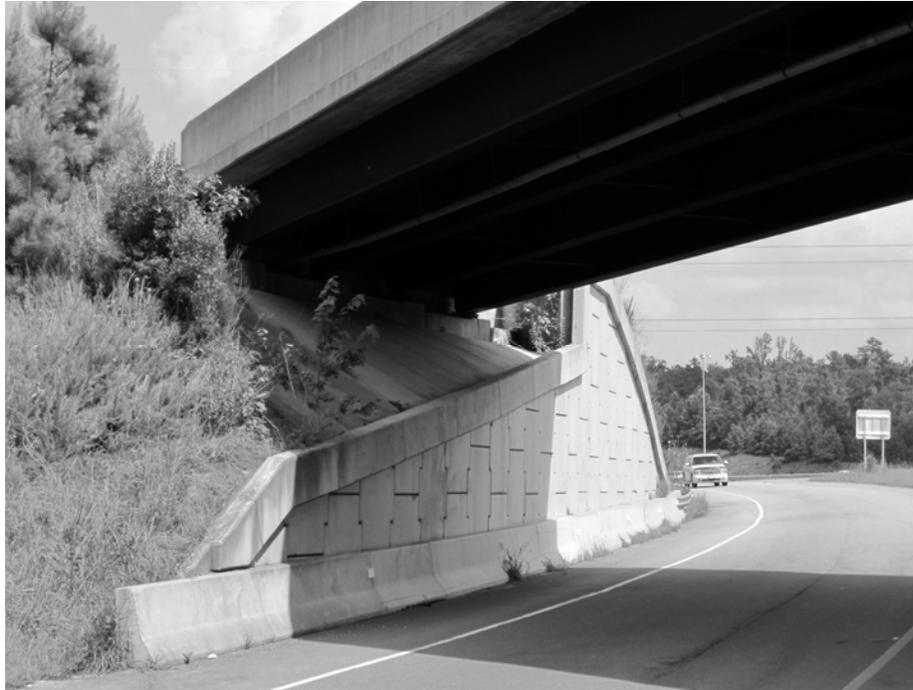
**Figure 48** A steel girder bridge where a small mechanically stabilized earth (MSE) retaining wall was used to reduce the severity of skew without significant increase in span length.
