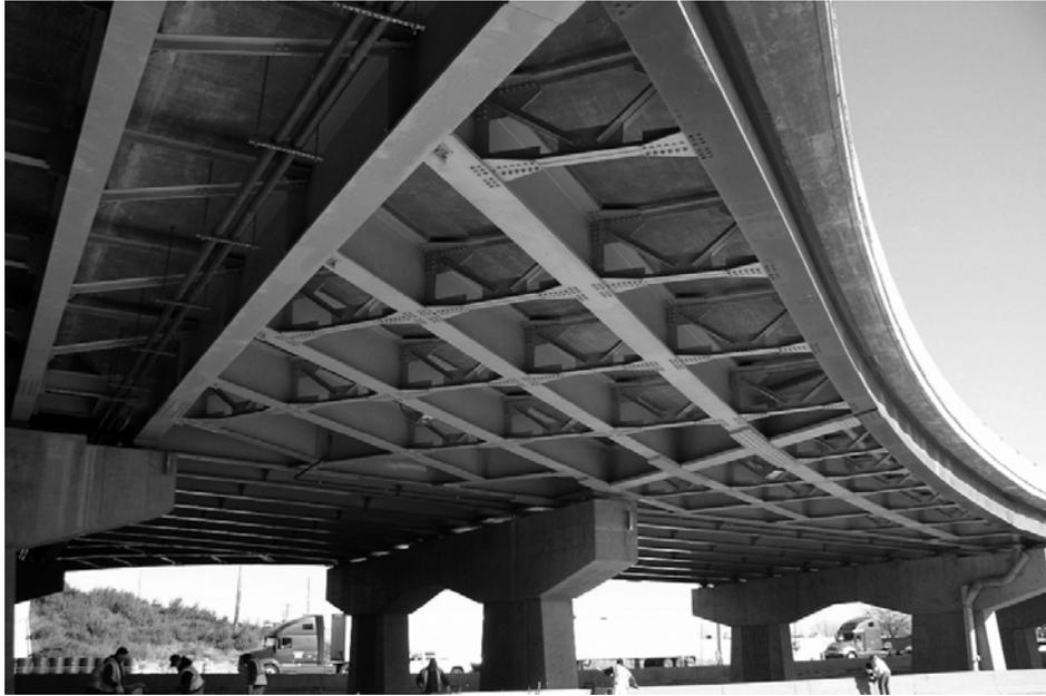
**Figure 62** View of curved infill framing area between two orthogonal regions of conventional parallel stringer framing in one of the ramp flare areas of a SPUI bridge structure.
