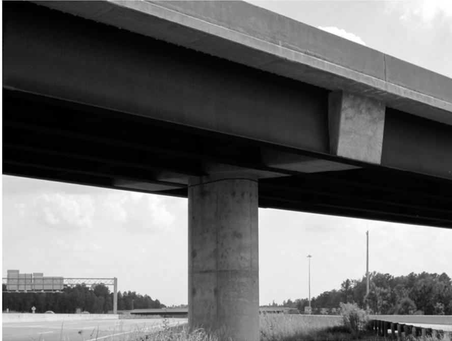
**Figure 50** An integral post-tensioned concrete pier cap used in an interchange in Raleigh, NC to avoid a conventional concrete rectangular cap (concrete drop cap). This allows the use of a radial cap while still maintaining adequate vertical clearances over traffic below the bridge.
