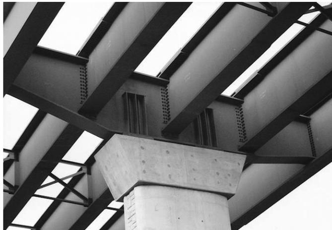
**Figure 49** An integral steel pier cap used to avoid a conventional concrete rectangular cap (concrete drop cap). This allows the use of a radial cap while still maintaining adequate vertical clearances over traffic below the bridge. This is a single steel pier cap; some designers and some owner-agencies prefer using a double I-beam cap to address redundancy issues.
