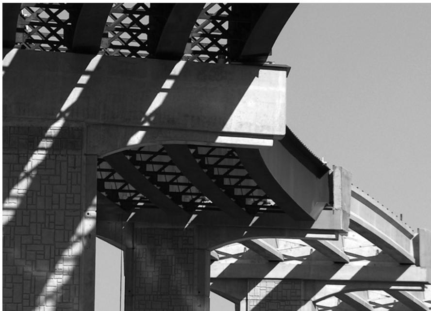
**Figure 51** Dapped ends on curved steel plate girders resting on an inverted-tee bent cap on a bridge in Texas. In this case, the dapped girder ends were used to match the depth of the precast girders in the next span but this same concept could be used to allow use of a radial bent cap the same depth as the girders, providing an effect similar to that of an integral bent cap.
